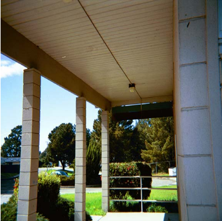
Figure 10: Glu-Lam Beam at Front
